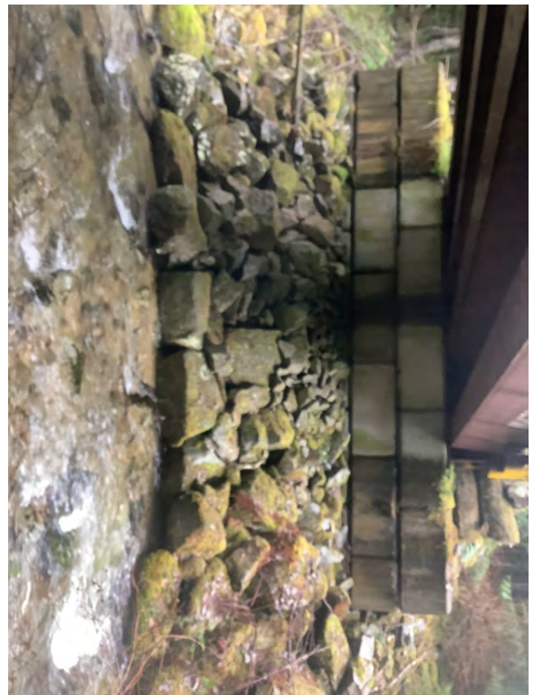
Right Bank Abutment when facing downstream
