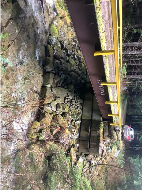
Right Bank Abutment when facing downstream
